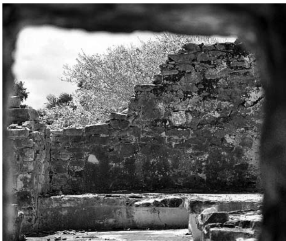
Figure 6: Tulum, Structure 25, looking west through the aperture in the east wall of Room A
