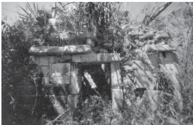
Figure 1. Chunchimai, Group 3, Structure 1, eastern façade with the entrance.
